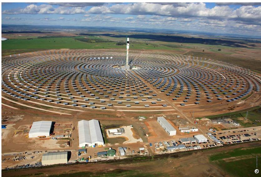
**Fig. 10.** The 19.9-MW<sub>e</sub> Gemasolar power tower with 15 h of molten-salt storage. (Photo: Torresol Energy, December 2010.)
