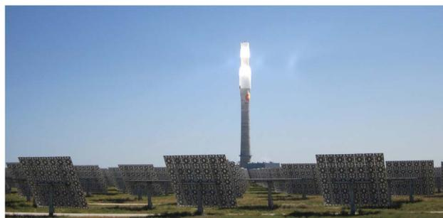
**Fig. 12.** The Gemasolar power tower in solar collection mode (daytime) with the molten-salt heated at the illuminated receiver. The support structures of the heliostat mirrors are also clearly shown. (Photo: Torresol Energy 2011.)
