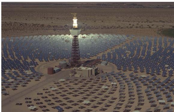
**Fig. 3.** The 10-MW<sub>e</sub> Solar Two power tower near Barstow, CA, which featured 3 h of molten-salt storage, and operated from 1996 to 1999. The receiver can be seen glowing white, indicating that the plant is operating in solar collection mode (daytime). (Photo: Sandia National Laboratories.)
