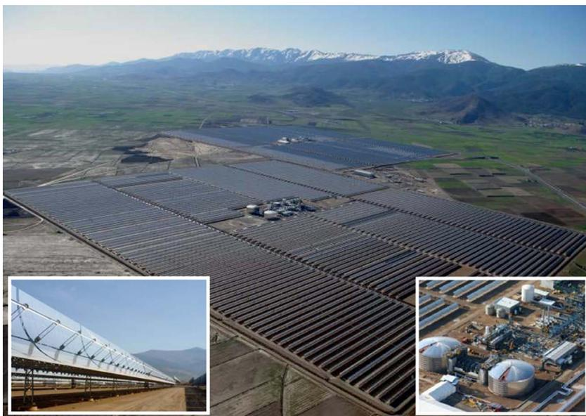
**Fig. 1.** An aerial view of the Andasol-1 and Andasol-2 plants (Photo: Cobra Energía). Left inset: Parabolic troughs tracking the sun at Andasol-1 (Photo: Author). Right inset: The hot and cold salt tanks and power block during construction of Andasol-1 (Photo: Cobra Energía).
