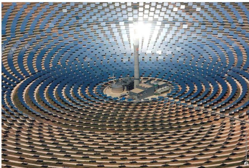
**Fig. 2.** The 19.9-MW<sub>e</sub> Gemasolar power tower with 15 h of molten-salt storage. (Photo: Torresol Energy, 2011.)
